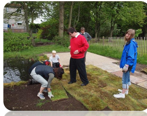
Putting finishing touches to the pond at Kilmaron School
